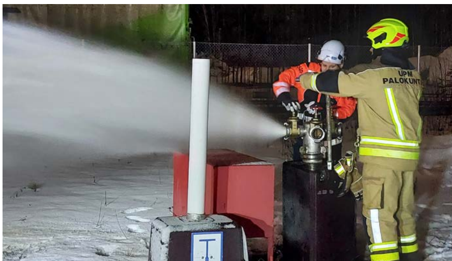
The mill's fire brigade checks the hydrants regularly.
